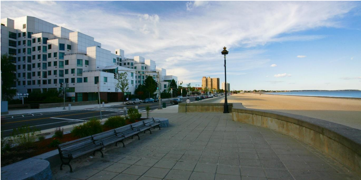
Hebrew SeniorLife's Jack Satter House (left), which recently received a HUD grant for efficiency and climate resilience. Source: Hebrew SeniorLife.
